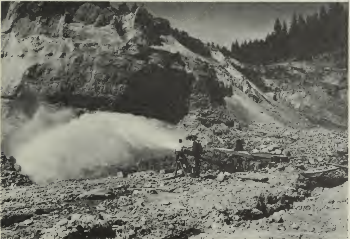
B, HYDRAULIC MINING AT RELIEF HILL, NEVADA COUNTY This is one of the few hydraulic mines to produce gold on a considerable scale in recent years. Such mines by Federal law must operate behind debris dams to restrain the tailing in the drainage basins of the Sacramento and San Joaquin Rivers. Photography, 1949; courtesy Thomas F. Ryder.
